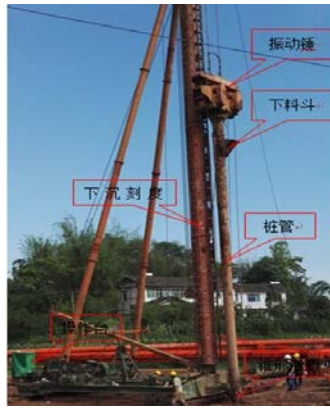
Fig.1. Drawing of traditional gravel pile machine
